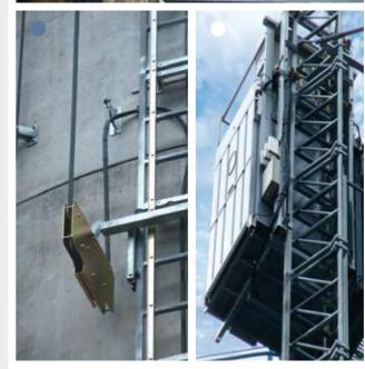
One- to four-sided closed base enclosure with tested landing door.
